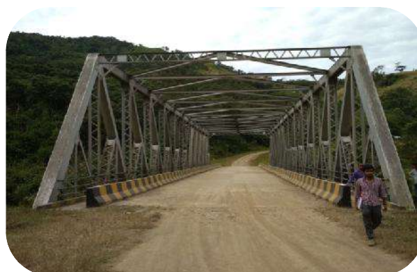
Existing Steel Truss Bridge at Ch-109.735 km
