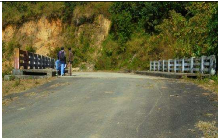
RCC T-Girder Bridge (Ch-76.081 km)
