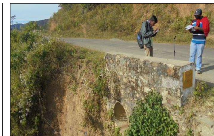
Culvert Inventory at Ch. 1+905 km
