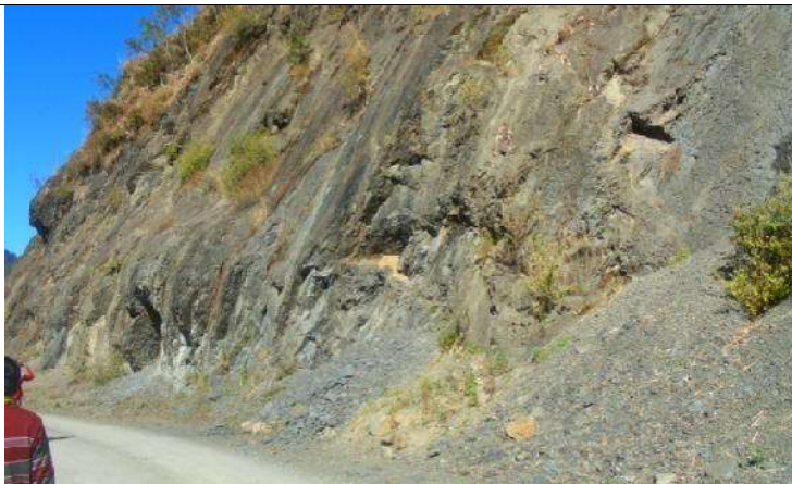
Hard Rock Zone (Ch-78.000 km)
