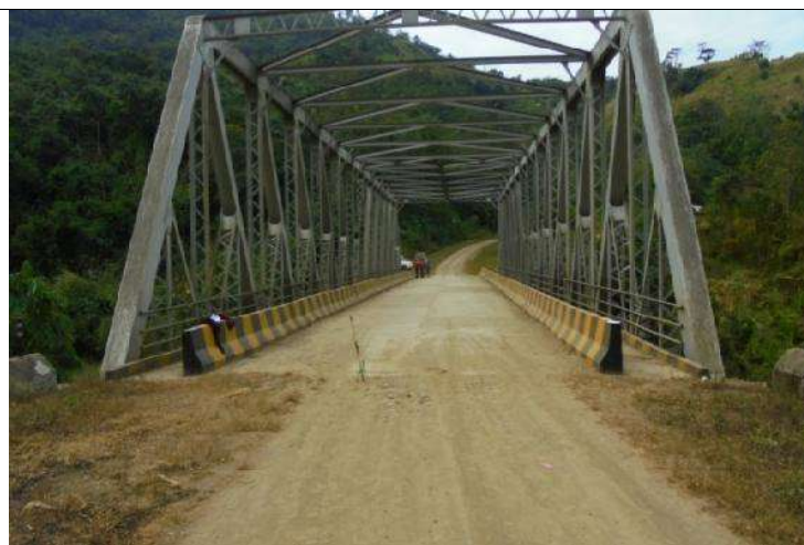
Dzuku Bridge (Ch-106.090 km)
