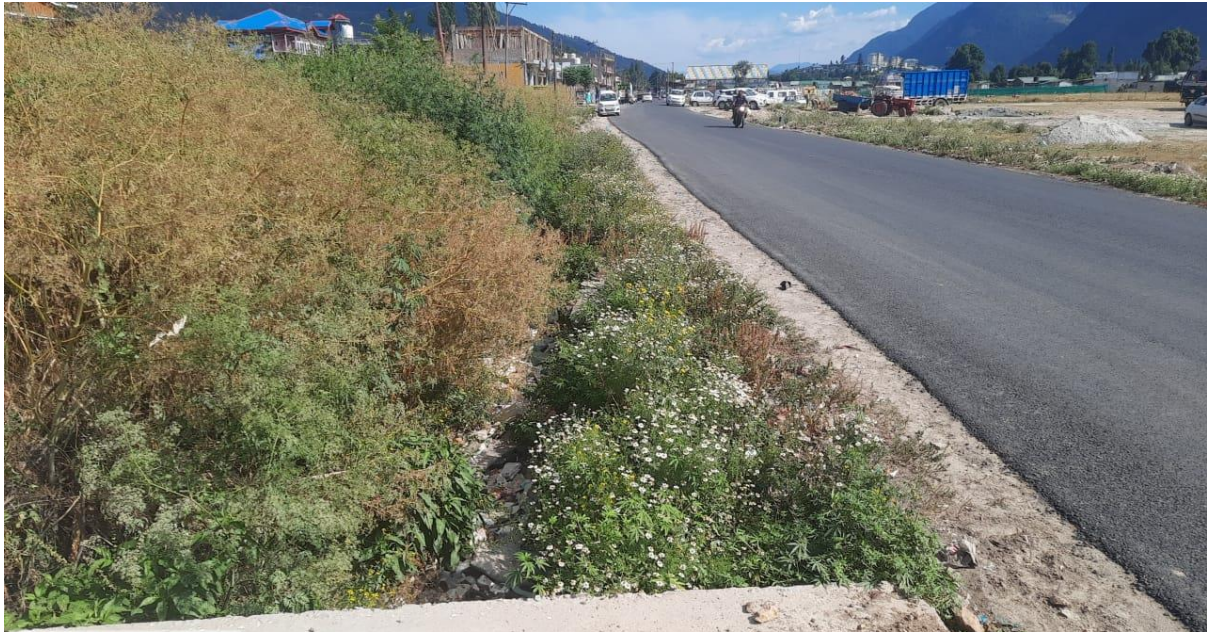
Time: 24-06-2021 15:51 Note: Damaged and Choked existing drain
