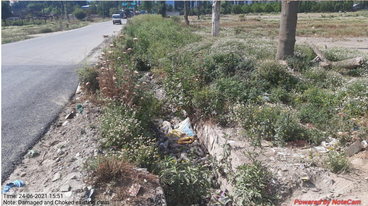
Time: 24-06-2021 15:51 Note: Damaged and Choked existing drain
