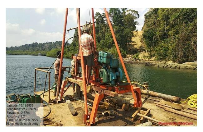
Fig.2. Sub Soil Investigation being Carried out at Baratang (Marine Borehole)
