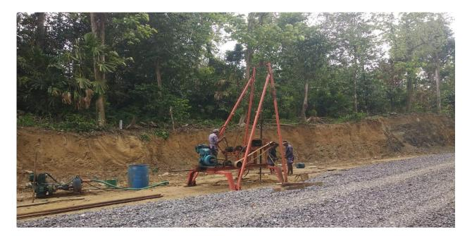
Fig.1. Sub Soil Investigation being Carried out at Baratang (Land Borehole)
