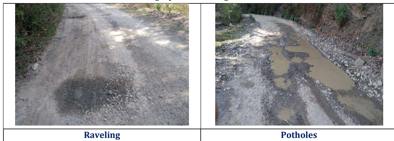
Plate – 2.2: Photographs of existing Pavement Distresses
