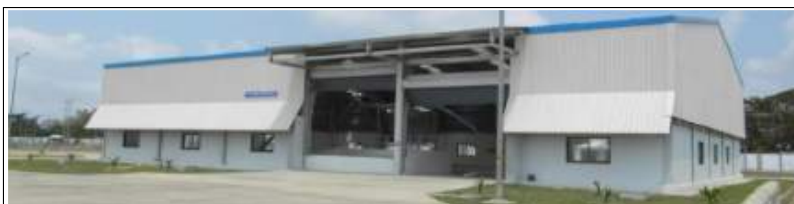
Typical Covered Sheds
