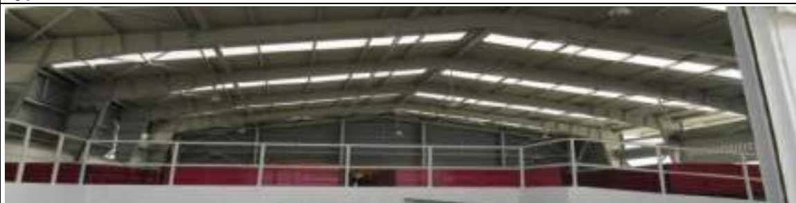
Typical Inside view of the Covered Shed
