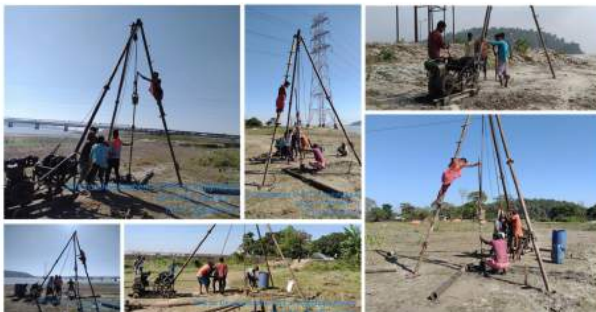
Figure 3.18: Selected Photographs – Geotechnical Investigations
