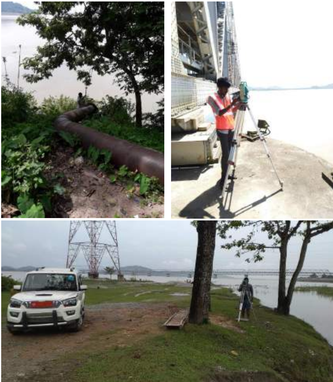
Figure 1.2: Selected Photographs – Topographic Survey
