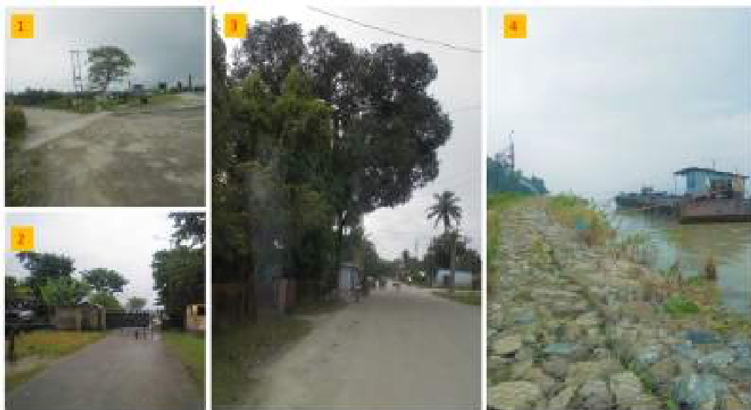
Figure 2.1: From Left to Right: 1 (NH-17 Crossing Towards IWT Site), 2 (IWT Gate), 3 (Approach Road) & 4 (Pontoon at Site)
