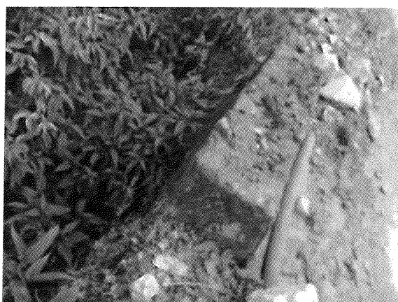
OFC Cable alongside Road
