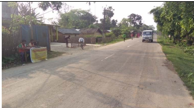
CTVC Survey near Lankeswar (Ch. 214.000 km)
