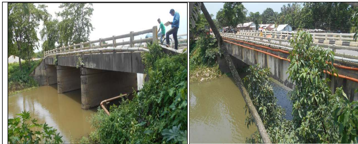
Plate 3.1.9: Photographs of Some Existing Minor Bridges
