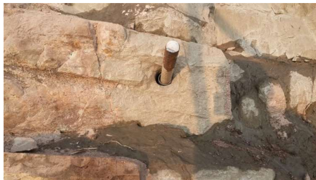
Figure 5: Centralizers at the outer end of nail
