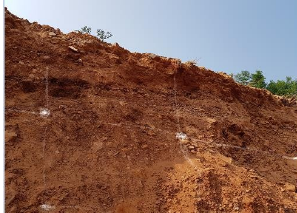
Figure 1: Marking of drill locations on the slope
