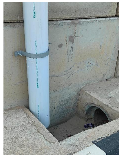
Takedown pipe at interval with 300mm Dia. HP in separator and cross connection to side drains.
