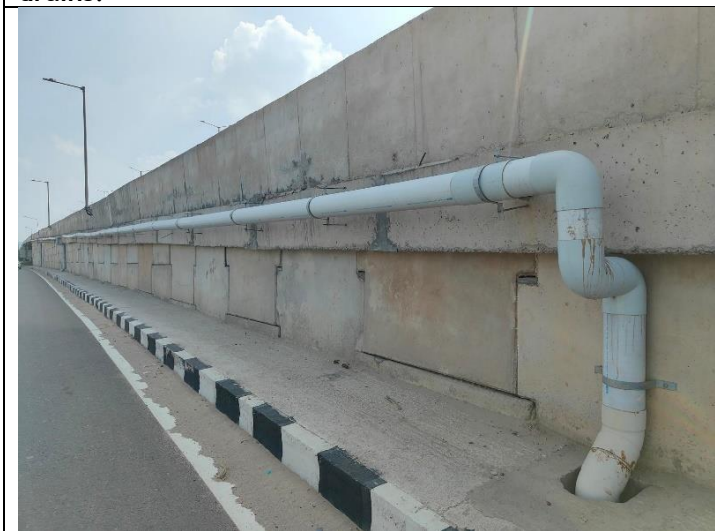
Alternatively: Long pipe slopped along ramp with connection with drainage spout & vertical take down pipe and connected to main drain
