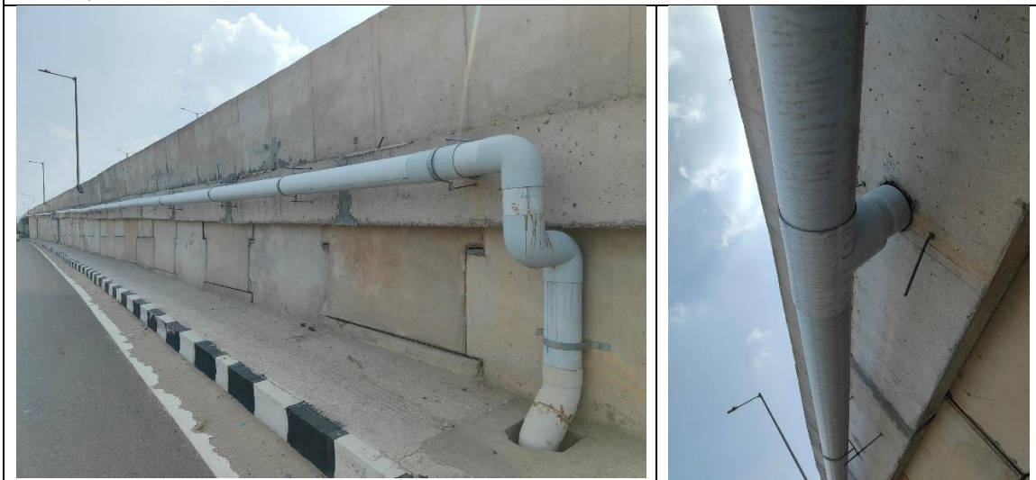
Alternatively: Long pipe slopped along ramp with connection with drainage spout & vertical take down pipe and connected to main drain
