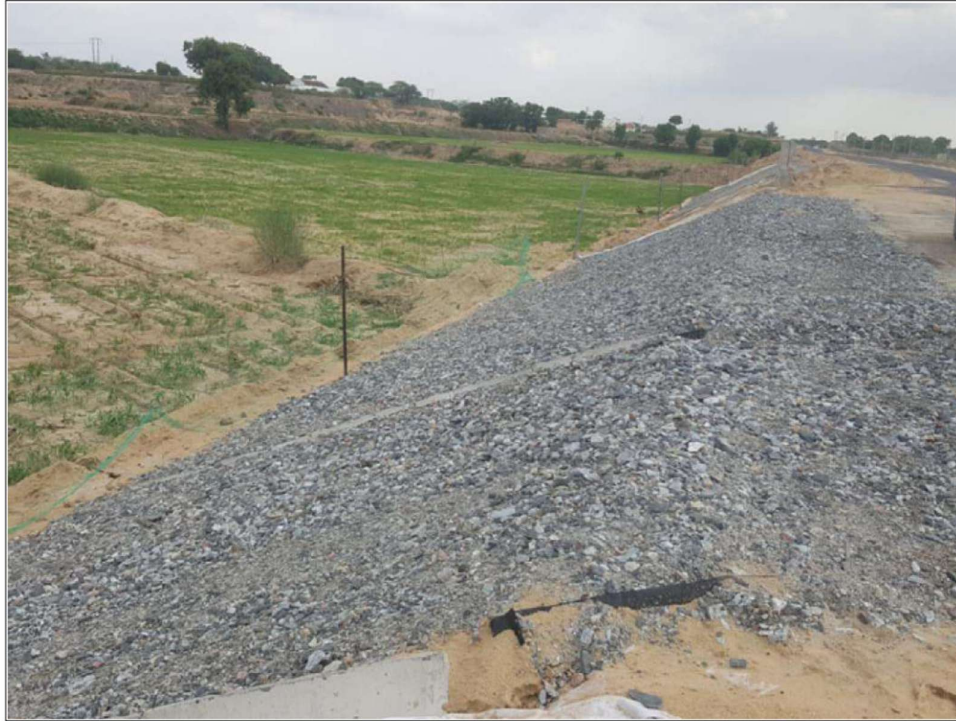
Slope is ready and filled with GSB
