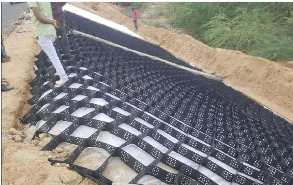
Installation of Geocell
